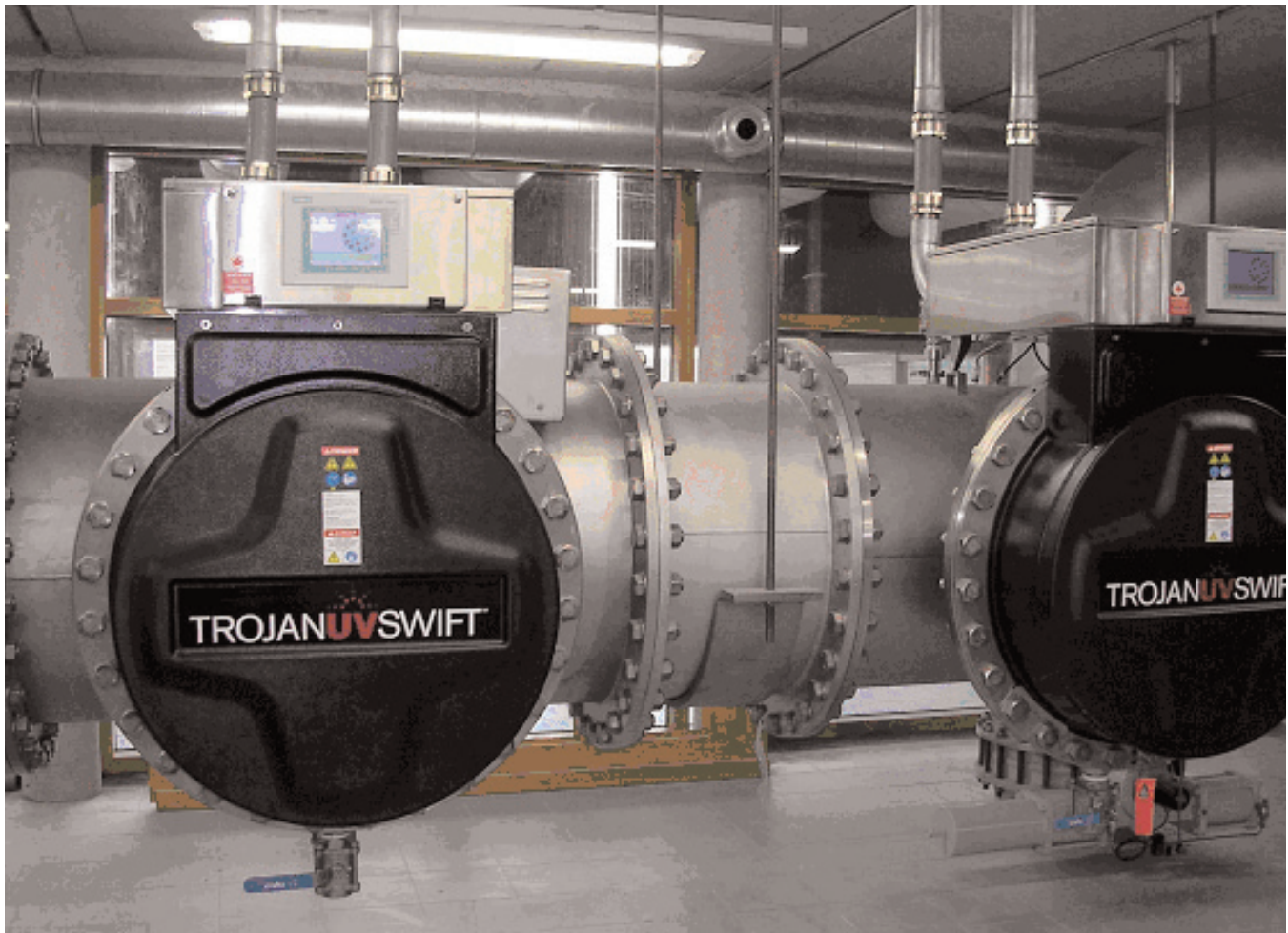
Figure 4: UV reactors in the full scale UV/H 2 O 2 system at the Andijk WTP.
