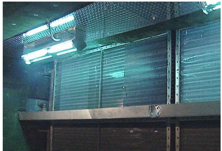
**Figure 2: Air disinfection system installed above cooling coils to provide simultaneous air and surface disinfection. Photo provided by Immune Building Systems, Inc. of New York.**
